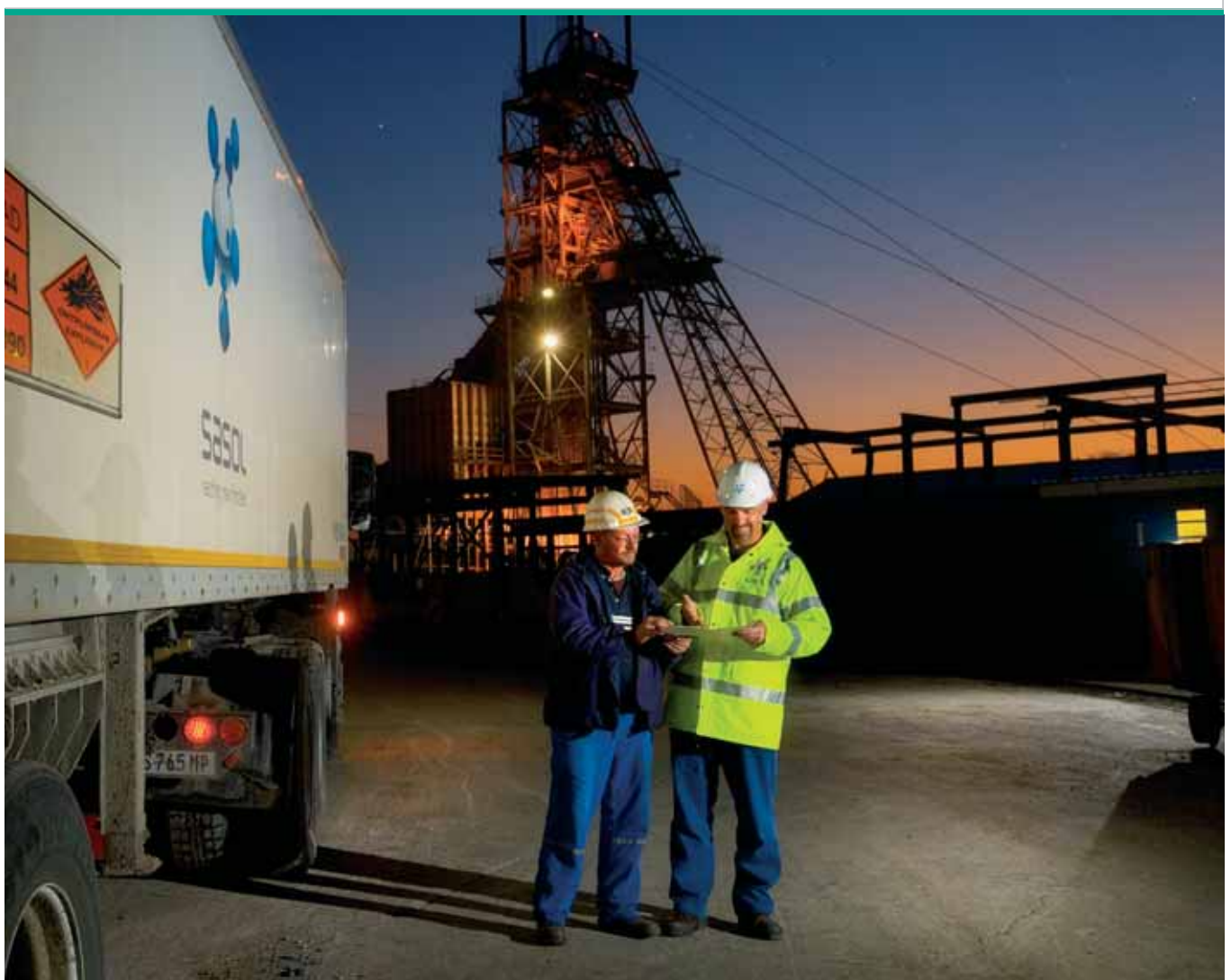
Sasol Nitro's product loading and off-loading facility at its plant in Rustenburg, as part of the new de-bottlenecking project.
