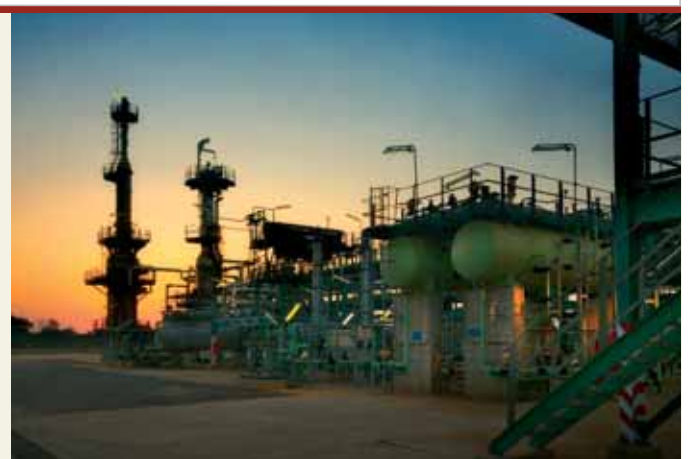
Central processing facility at Temane in Mozambique.
