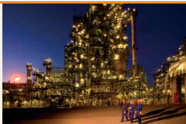
The selective catalytic cracker at Secunda recorded significant gains in availability and stability.
