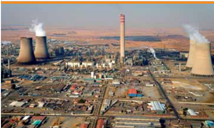
The maintenance shutdown of our main facilities at Secunda went smoothly.
